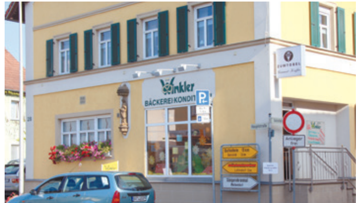
View of the headquarters where production also takes place.
