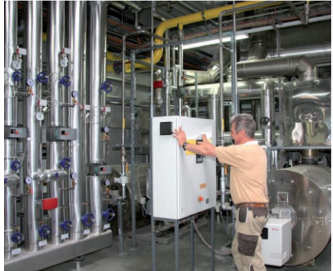
Recovered heat from ovens and refrigeration systems is fed to the building's hot water supply.
