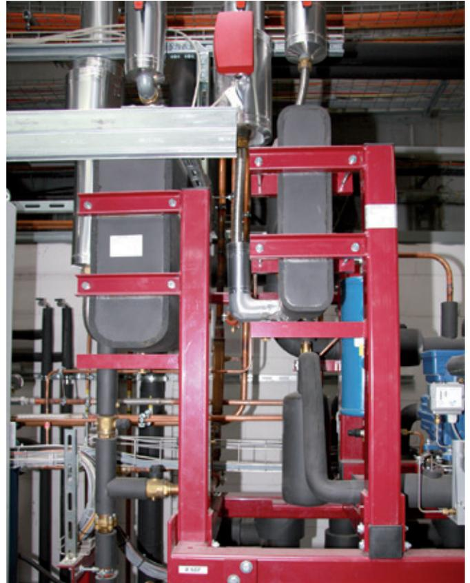
Detailed view of the refrigeration system with the plate heat exchangers.
