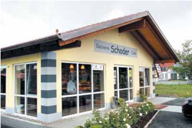
The Schoder family financed the construction of an additional building for the new branch outlet in Untermerz bach.
