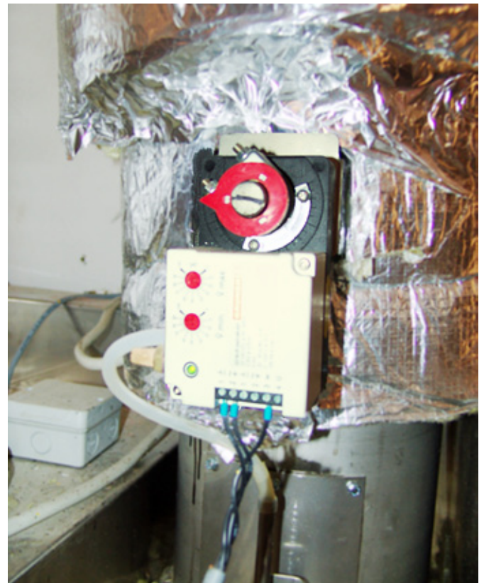
Technology in detail: actuator for the innovative and dynamic draught regulating valve.
