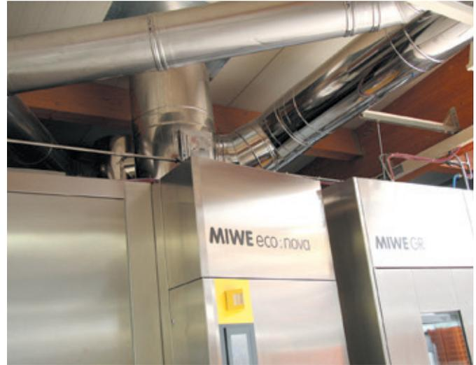
Detailed view of the eco:nova: a pipe for flue gas and a pipe for steam coming from the ovens.
