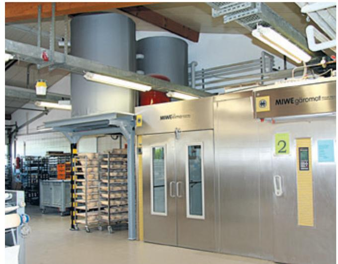
The accumulators were installed on a raised floor so that no space was wasted in the bakery.
