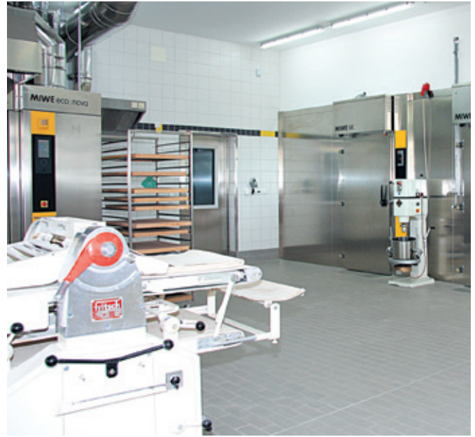
View of the refrigerating unit.
