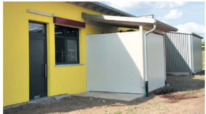
Outside view of the TLK. The floor plate for the GVA has already been laid.
