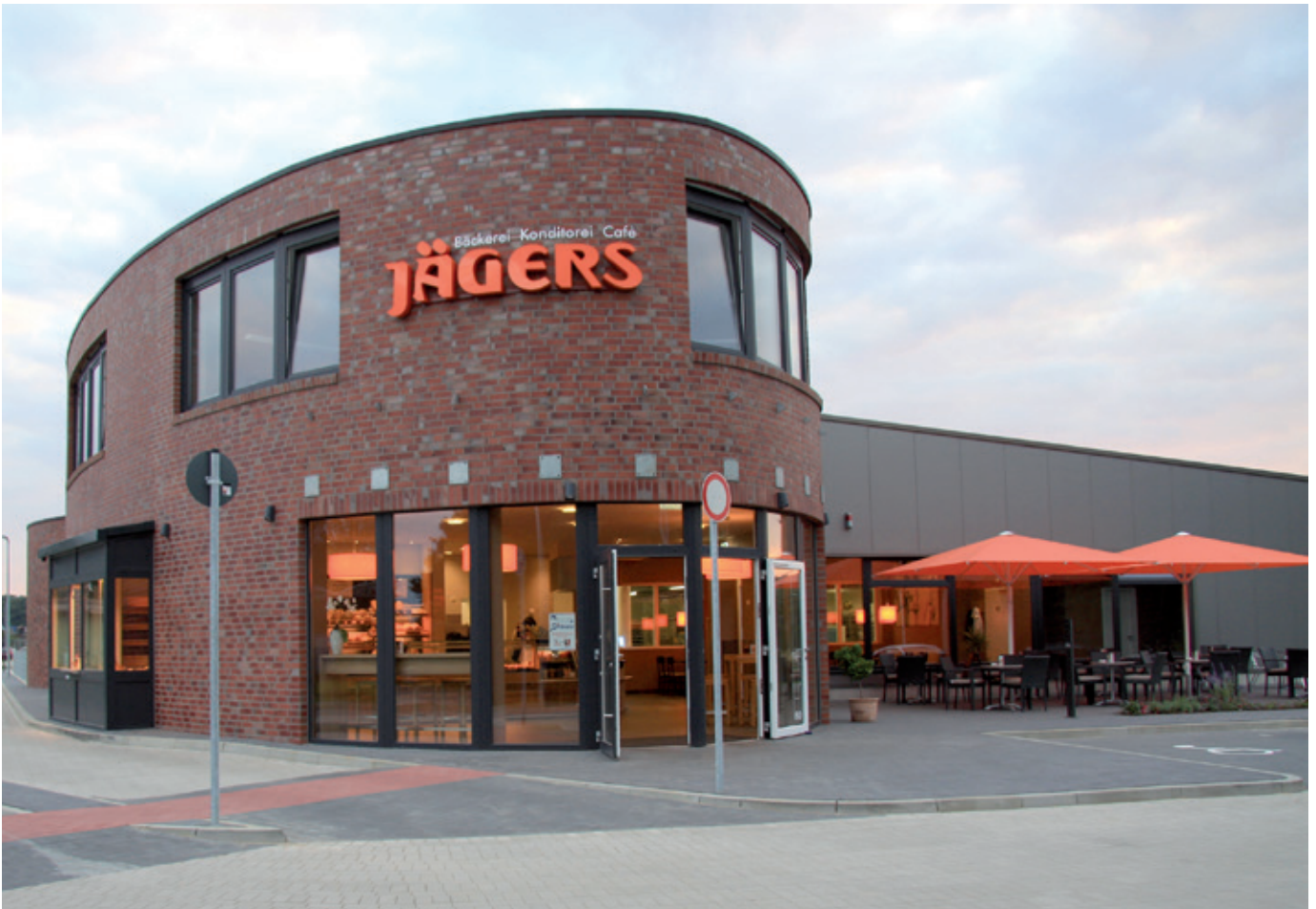
The Jägers building is located directly on a popular main road through town. It really stands out, just like the company's energy concept.
