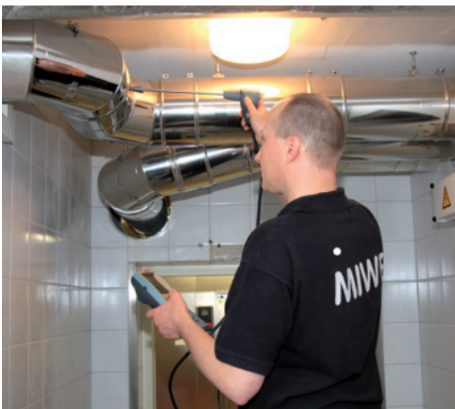
MIWE employee performing the waste gas measurement in accordance with DIN 8766.
