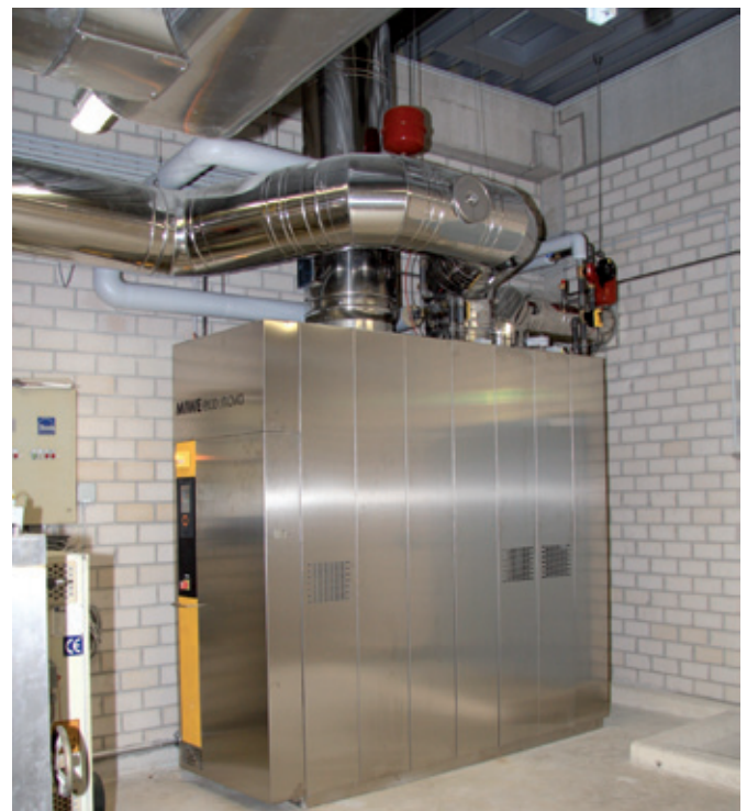
One MIWE eco:nova is supplied by flue gas from the central heating boiler for the thermal oil ovens. It is located directly beside the central heating boiler.
