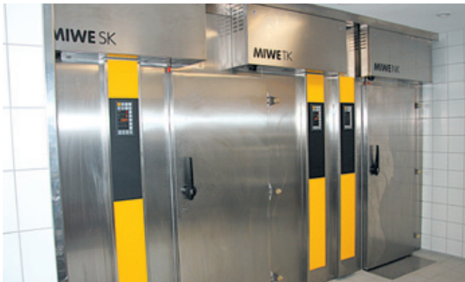
Nowadays, a bakery requires the implementation of refrigeration technology. The onsite equipment includes cooling cells for cream products (MIWE SK), a freezer storage unit (MIWE TK) and a cold storage unit (MIWE NK).
