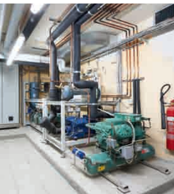
Here too, a large amount of heat is recovered thanks to the MIWE eco:nova. The engineering room contains a compound refrigeration system with a buffer tank and specially programmed control unit.
