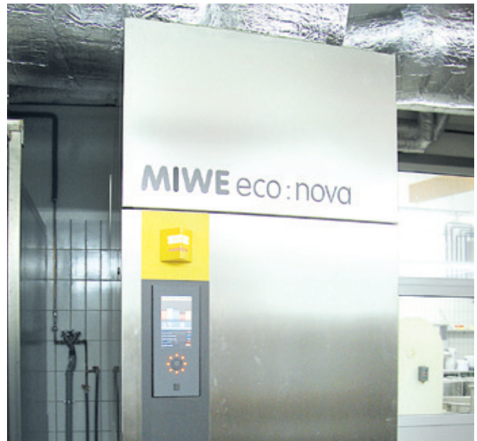
The heat recovery unit MIWE eco : nova is also controlled by means of Touch Control MIWE TC.
