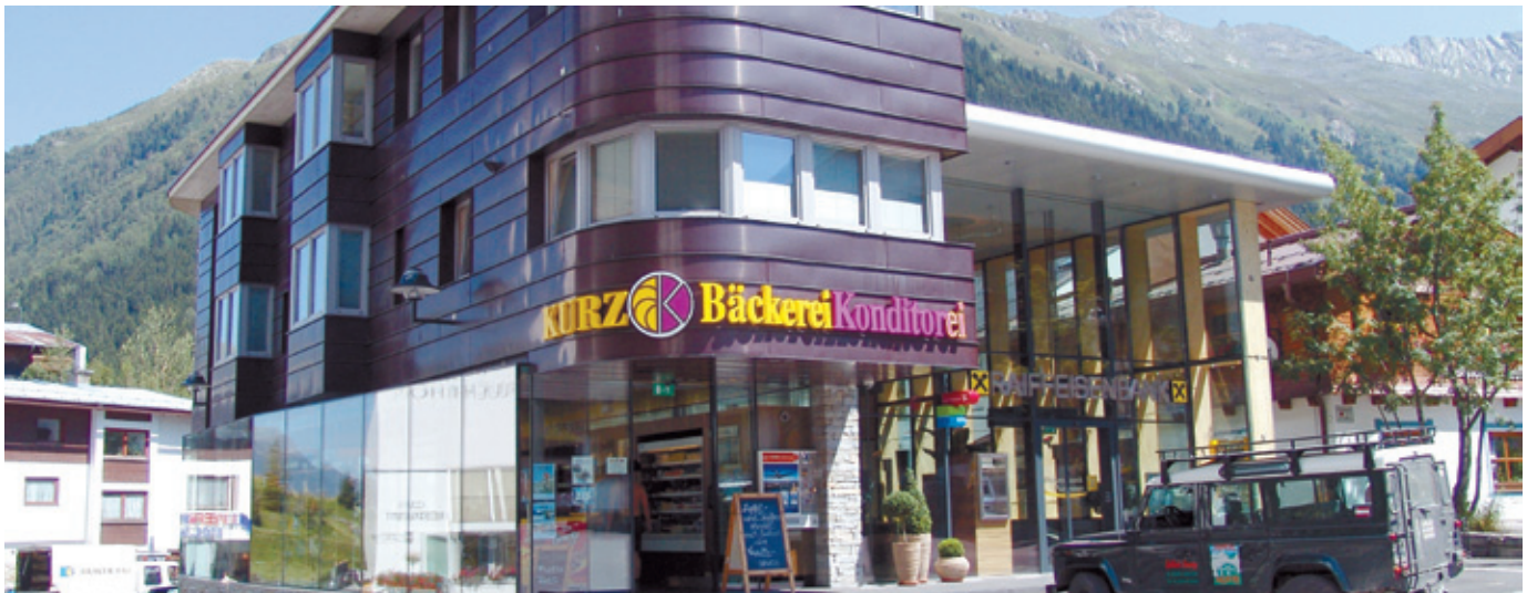
The new building for the branch outlet in Galtür, featuring an emergency bakery in the cellar, was built as a semi-detached house together with a bank.
